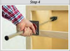
Making sure slide bracket is firmly attached to end of tool, carefully extend aluminum rod to back of cabinet with other hand.
