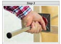
With your hand, grasp installation tool handle and place it in the bottom left corner of drawer opening. Be sure that the handle is flush and square against face frame.
